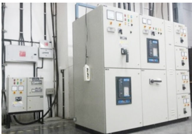
Figure A.2.7.2 Control panel for Power Supplies
